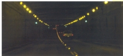
In-pavement centreline delineation
