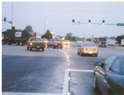
Delineated left turn at an intersection
