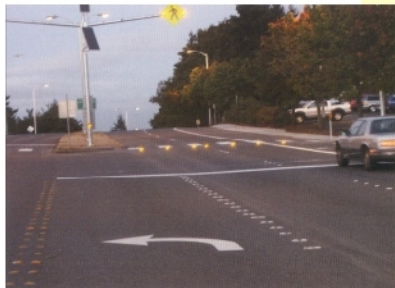
A solar-powered Smartstud ™ crossing system
